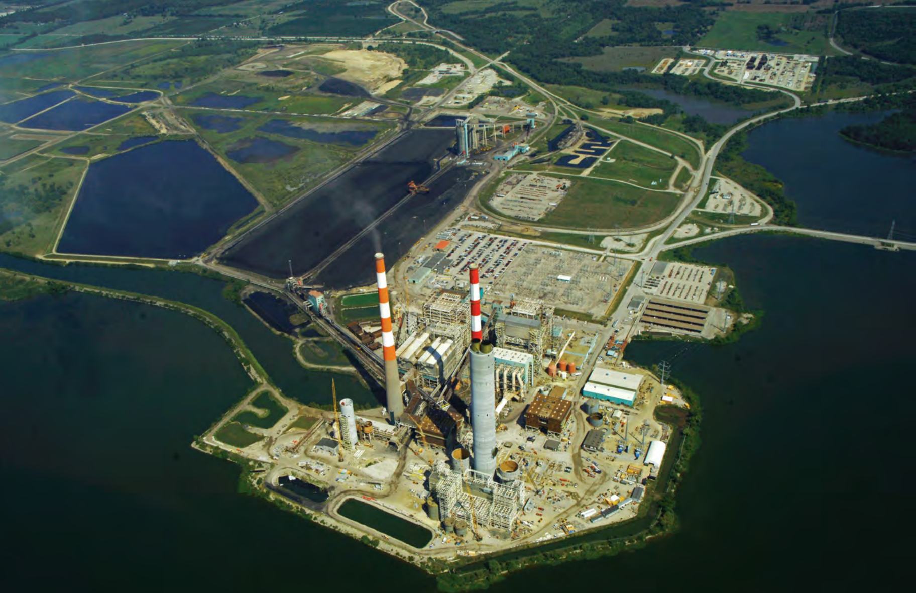
La Cygne Generating Station La Cygne, KS
